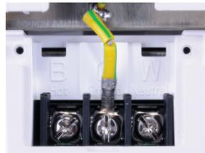
6. Unscrew the screws for the power terminal and connect the cables from the power source. Then tighten screws, ensure the wires are secured.
